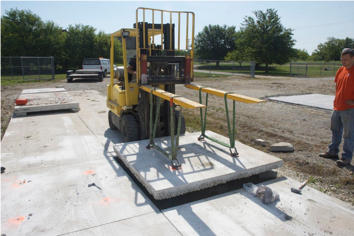
1.8m x1.8m slab size by 9cm thick
